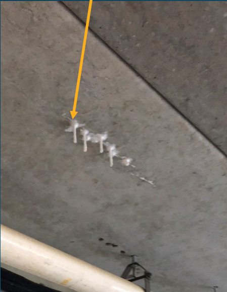
Efflorescence ("stalactites")
